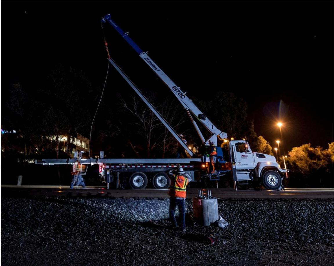
Construction to make Caltrain a modern, electric commuter rail system continues! This month, crews installed foundations, poles, and wire from South San Francisco to San Jose. Work was also performed on eight traction power facilities in San Francisco, South San Francisco, San Mateo, Redwood City, Palo Alto, Sunnyvale, and San Jose.
