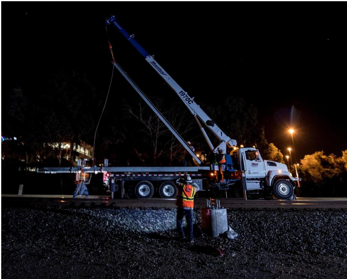
Construction to make Caltrain a modern, electric commuter rail system continues! This month, crews installed foundations, poles, and wire from South San Francisco to San Jose. Work was also performed on eight traction power facilities in San Francisco, South San Francisco, San Mateo, Redwood City, Palo Alto, Sunnyvale, and San Jose.
