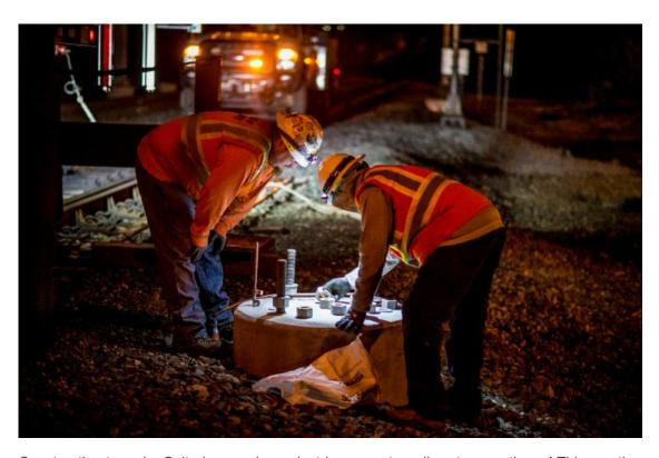
Construction to make Caltrain a modern, electric commuter rail system continues! This month, crews continued foundation installation from South San Francisco to Menlo Park and pole installation from South San Francisco to San Mateo. Five traction power facilities are currently under construction in South San Francisco, San Jose, Redwood City and San Mateo.
